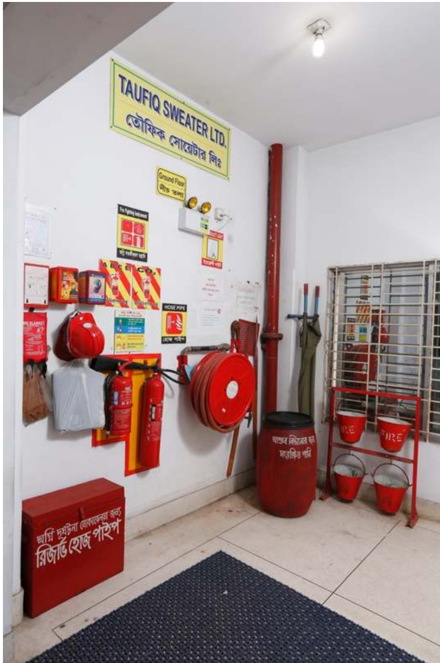
Fire Fighting equipments & Alarm Control Panel Health & Safety
