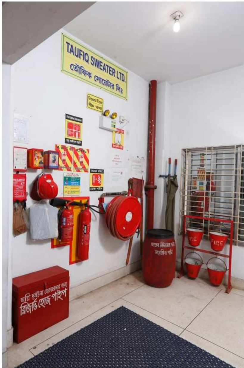
Fire Fighting equipments & Alarm Control Panel
