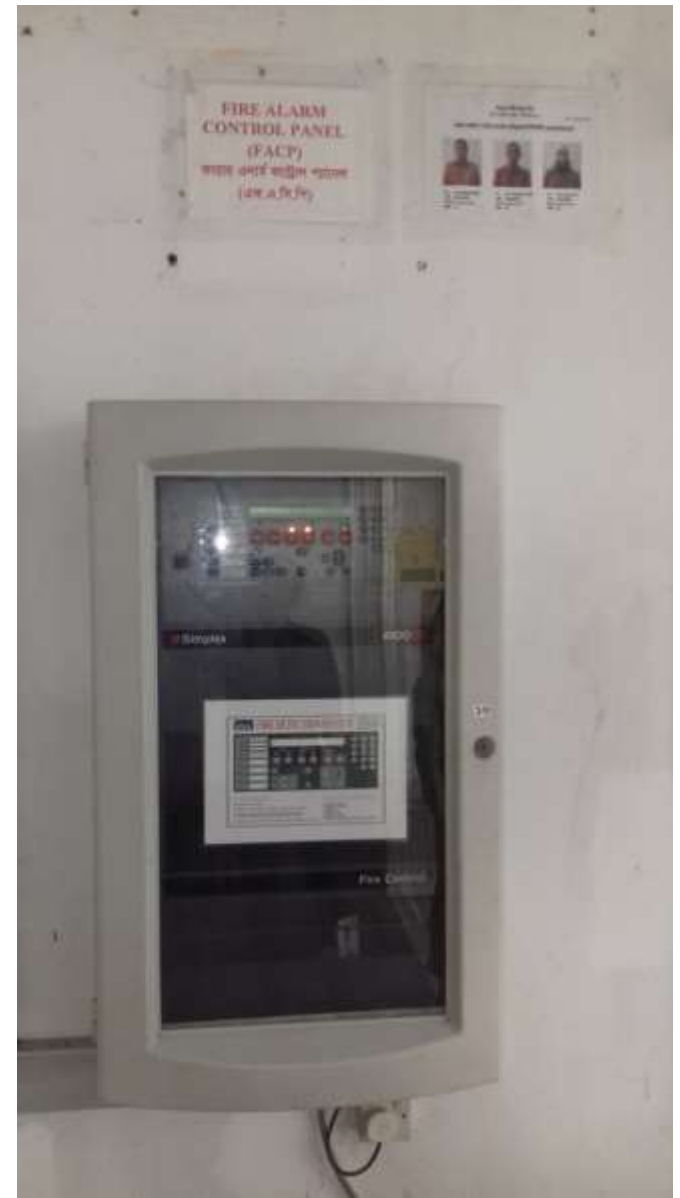
Fire Fighting equipments & Alarm Control Panel
